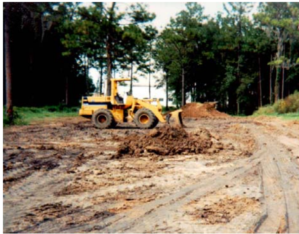
Figure 12. Tractor removing stockpiled soil materials for use in other areas.
